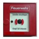
Smashing in the panel and pressing the button will directly alert the fire department and trigger an acoustic in-house fire alarm (alarm horn) in order to alert other persons in the building to the situation.
